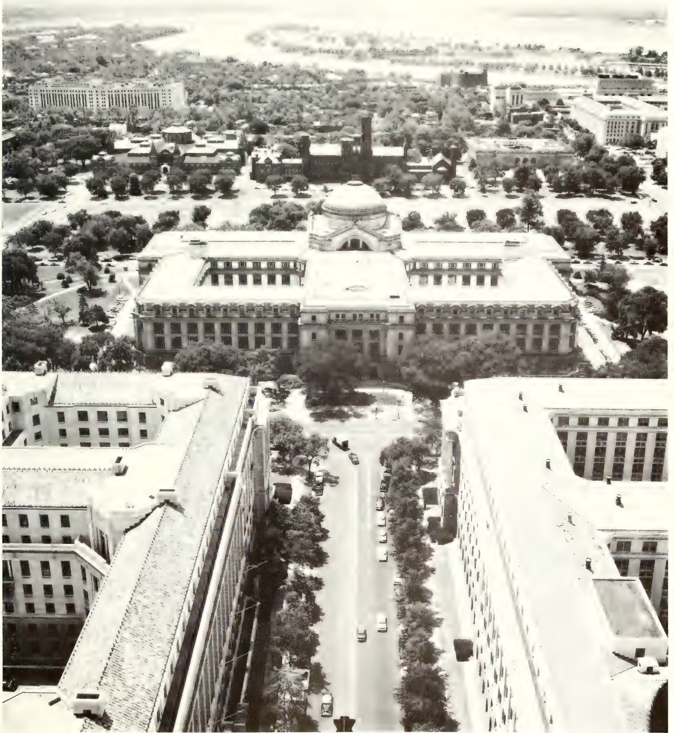
Aerial view looking south down Tenth Street, showing small parks on either side of the building, where the wings now stand. The projections on the south side, at the corner of each court, house the freight elevators. In the background are the Freer Gallery to the right of the Castle and the Arts
